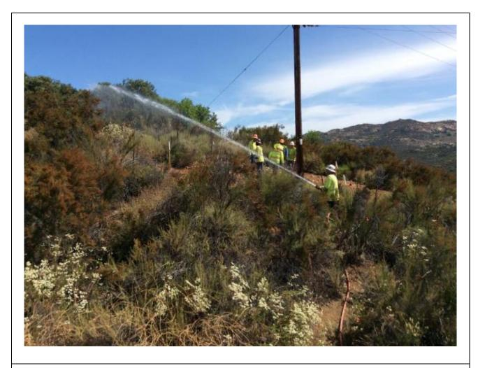
**Photo 6:** In preparation for vegetation at Pole Z272905 (TL 625C) to be chipped upon removal, the area was wet down prior to the activity in accordance with the CFPPP for the day's fire conditions (Elevated FPI off CNF land). A Fire Patrol was also present with at least 100 gallons of water and a complete set of fire tools on site.
