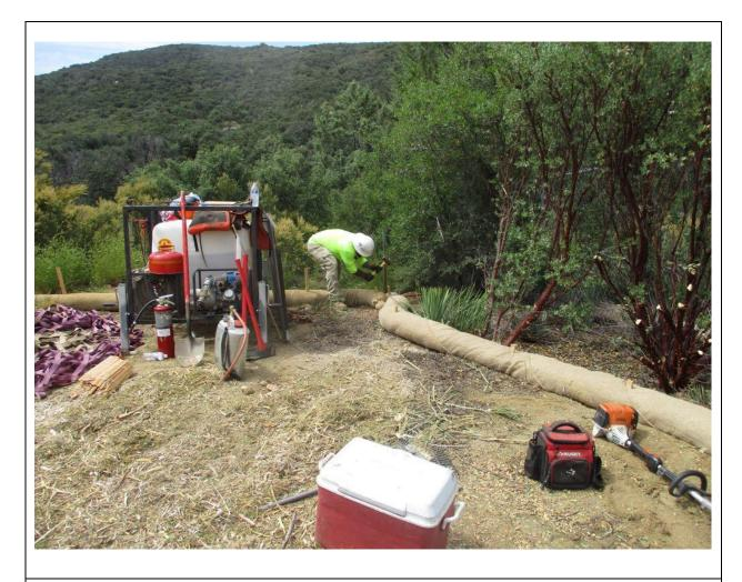
**Photo 2:** A construction worker observed installing perimeter fiber rolls at Pole Z173110 (TL 629A) for erosion control in accordance with the ECP and SWPPP (MM HYD-01, MM BIO-7).
