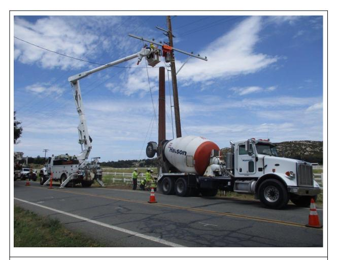
**Photo 1:** A construction crew was observed removing 12 kV wire protectors used during pole setting, and backfilling around the pole base with concrete on TL 629A. A crew member was conducting traffic control along Viejas Boulevard during the activities in accordance with the TCP (APM TRANS-05).
