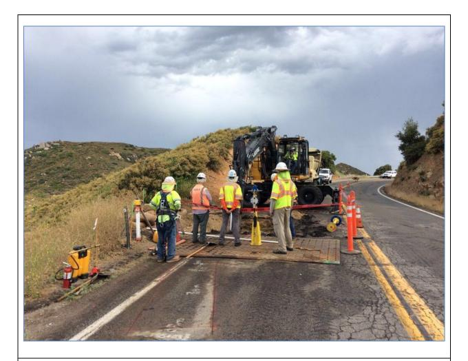
**Photo 4:** A biological, archaeological, and cultural monitor were present during vault excavation (C 440) in accordance with MM BIO-22, MM CUL-1, and APM CUL-04. A complete set of fire tools were staged on site (5-gallon backpack pump, round point shovel, Pulaski, and 2A10BC fire extinguisher) in accordance with the CFPPP (MM FF-1).
